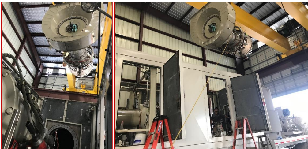
Figure 6. Engine lifting method.
